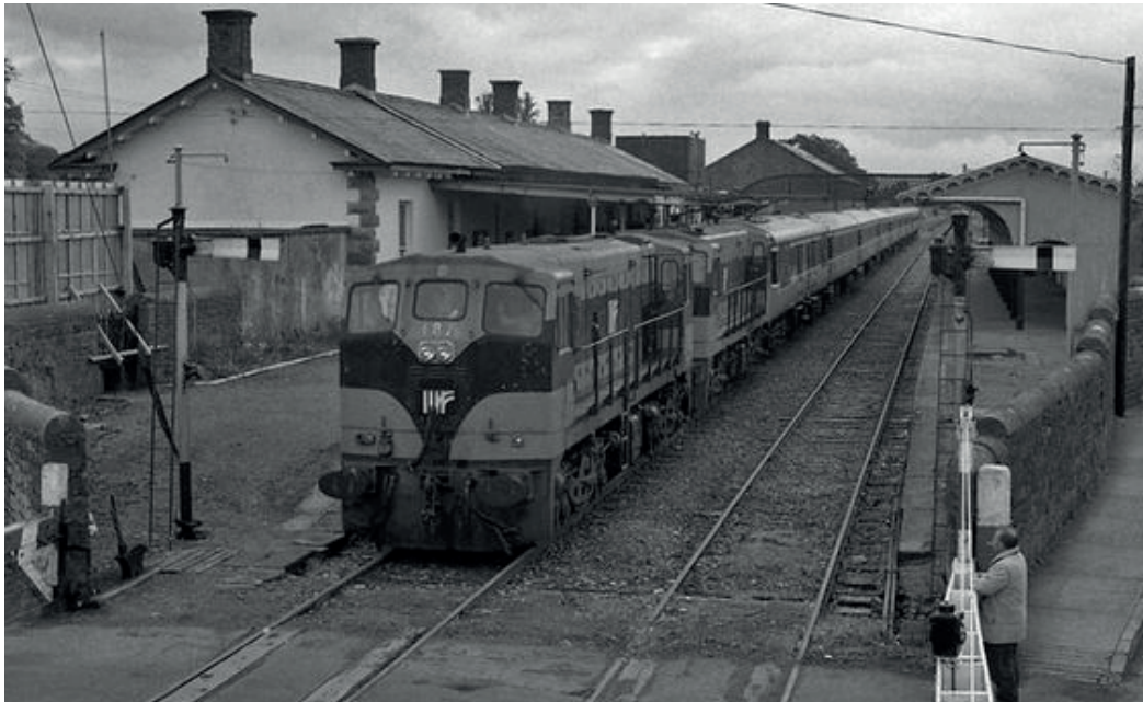
Former Railway Line
